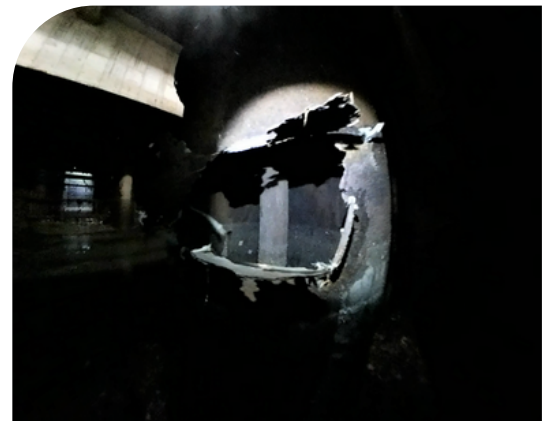
The 48" carbon steel pipe had 16"x35" corrosion holes that needed repaired.
