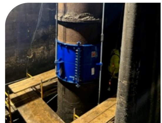
A Smith-Blair 675 Split Encapsulating Fitting was utilized to repair the holes.
