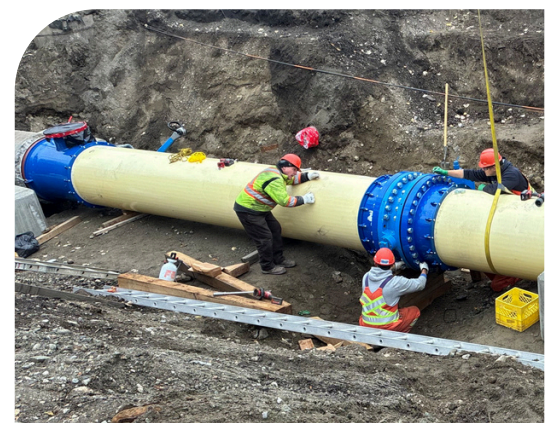
Smith-Blair 935 and 936 spigot adapters and two Smith-Blair 913 coupling assemblies were used on this project.
