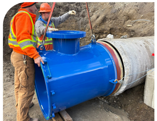
A Smith-Blair 936 is positioned into an existing bell.
