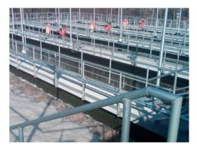
These seven deep bed filters are 89' long x 13' wide and provide Enhanced Nutrient Removal. Effluent nitrate is <0.5 mg/L and effluent phosphorus is <0.2 mg/L.
