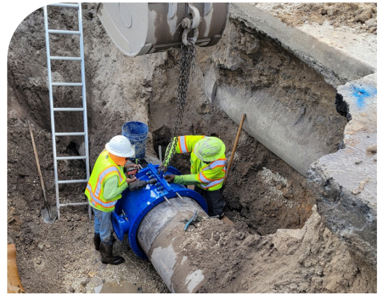
A crew works to install a Smith-Blair 624 MJ style tapping sleeve
