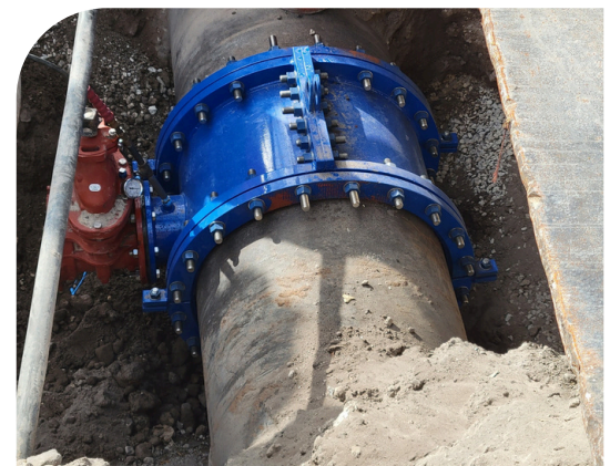
Custom Smith-Blair 624 MJ style tapping sleeve used on this project.
