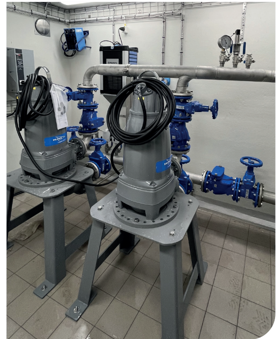
Dry-installed booster pumps in Granås that increase pressure and flow in the pressure main.
