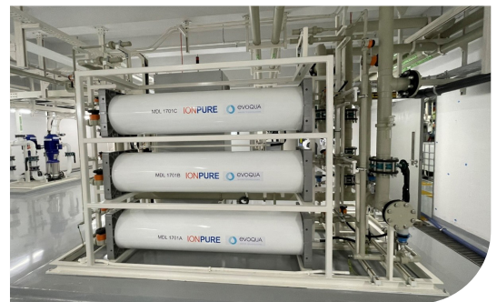
Multimedia filtration (Image 1) integrates with Vantage™ RO (left) and Ionpure® VNX Ultra CEDI (right) to deliver ultrapure water system.
