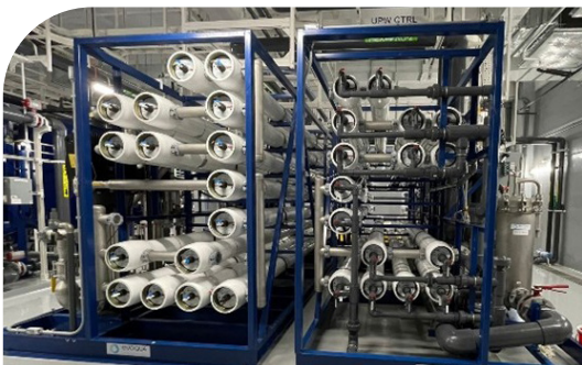
Multimedia filtration (Image 1) integrates with Vantage™ RO (left) and Ionpure® VNX Ultra CEDI (right) to deliver ultrapure water system.
