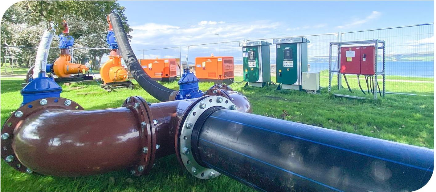
Delivering a resilient temporary pumping solution to maintain uninterrupted wastewater services during critical network infrastructure works.
