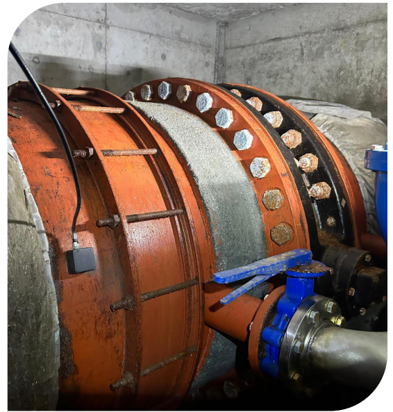
Tracking the free-swimming PipeDiver platform during the 7.7-kilometer inspection
