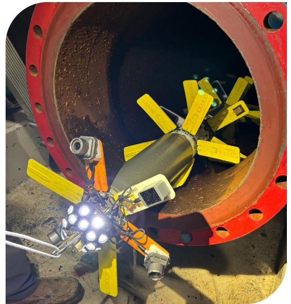
Launching the PipeDiver® platform from City of Kamloops' High Lift Station
