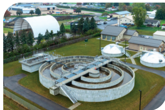
Aerial view of the Caledonia, MN Wastewater Treatment Facility
