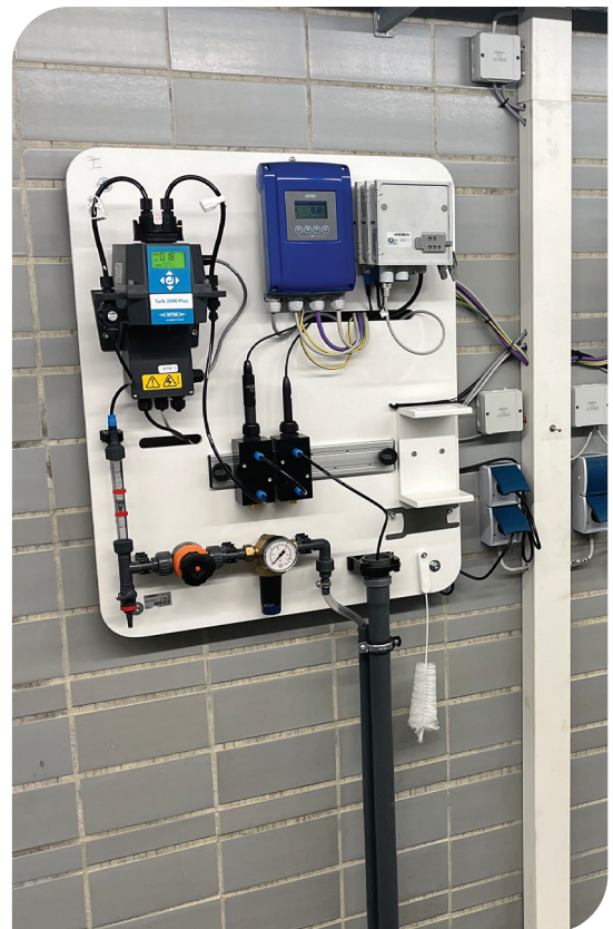
Fig. 2: WTW drinking water panel at the outlet of the gravel filter systems for monitoring turbidity, pH and oxygen
